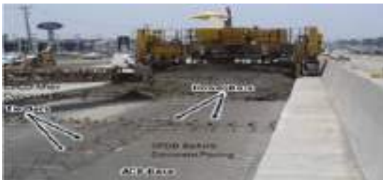
Fig. 7: Continuously Reinforced Concrete Pavement [21]
