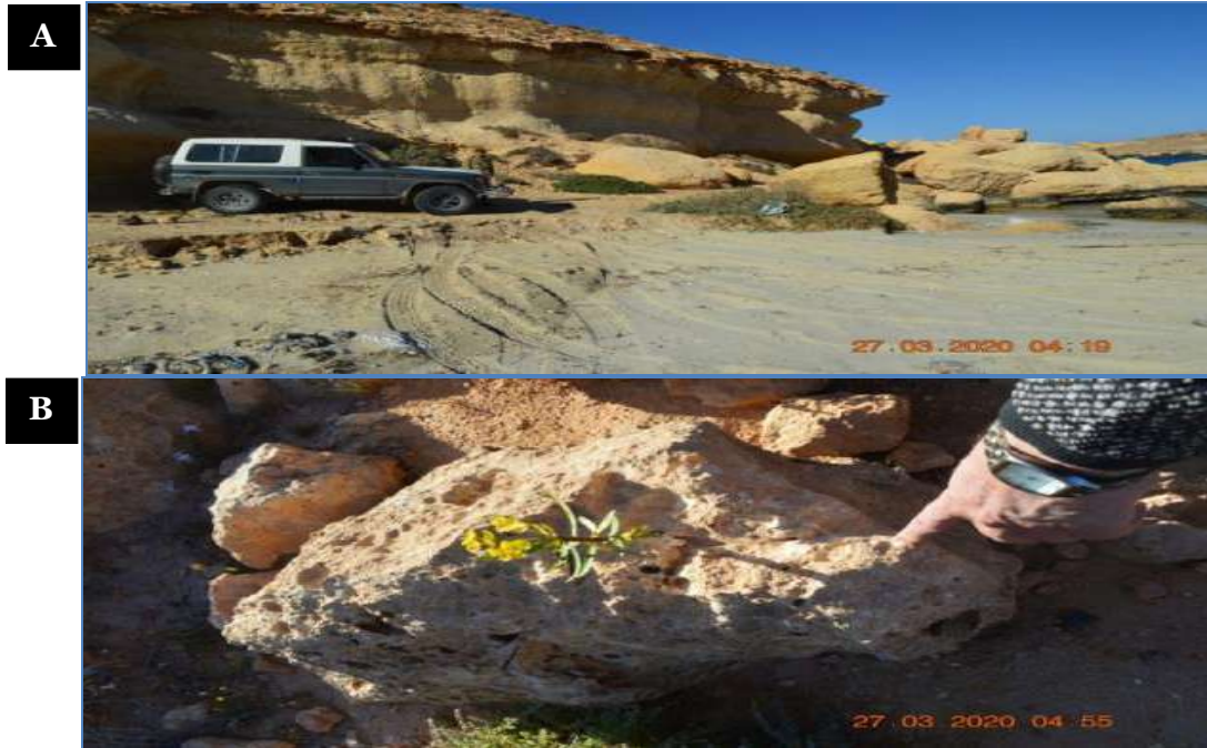
Fig. 18: Rock spreads and blocks slides: (A) Cliff failure; (B) Growing plant in boulder rock.
