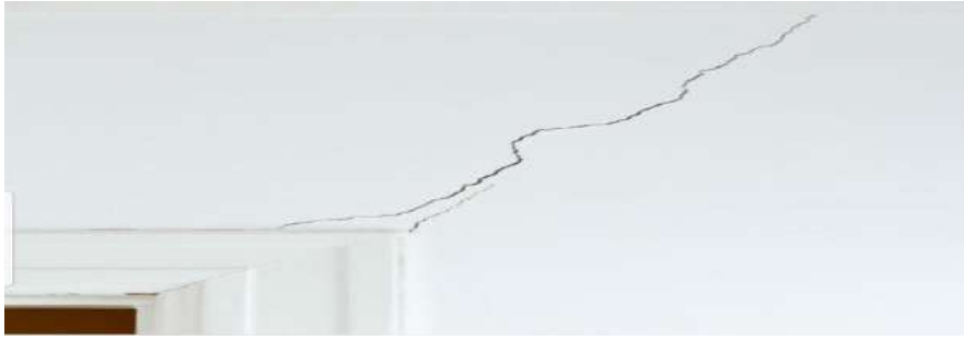
Fig. 3: shows the cracks at the top of the window
